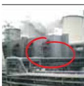
Damaged Insulation.
